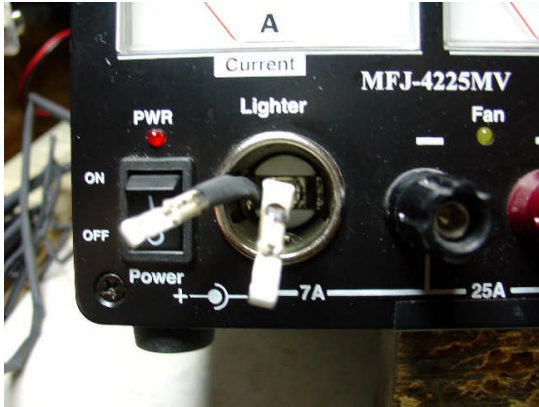
Braid assemblies soldered in place
